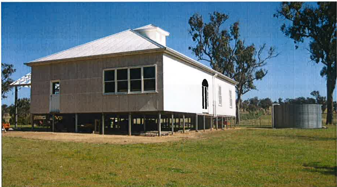
Photo 1: View of dwelling and water tank looking south
